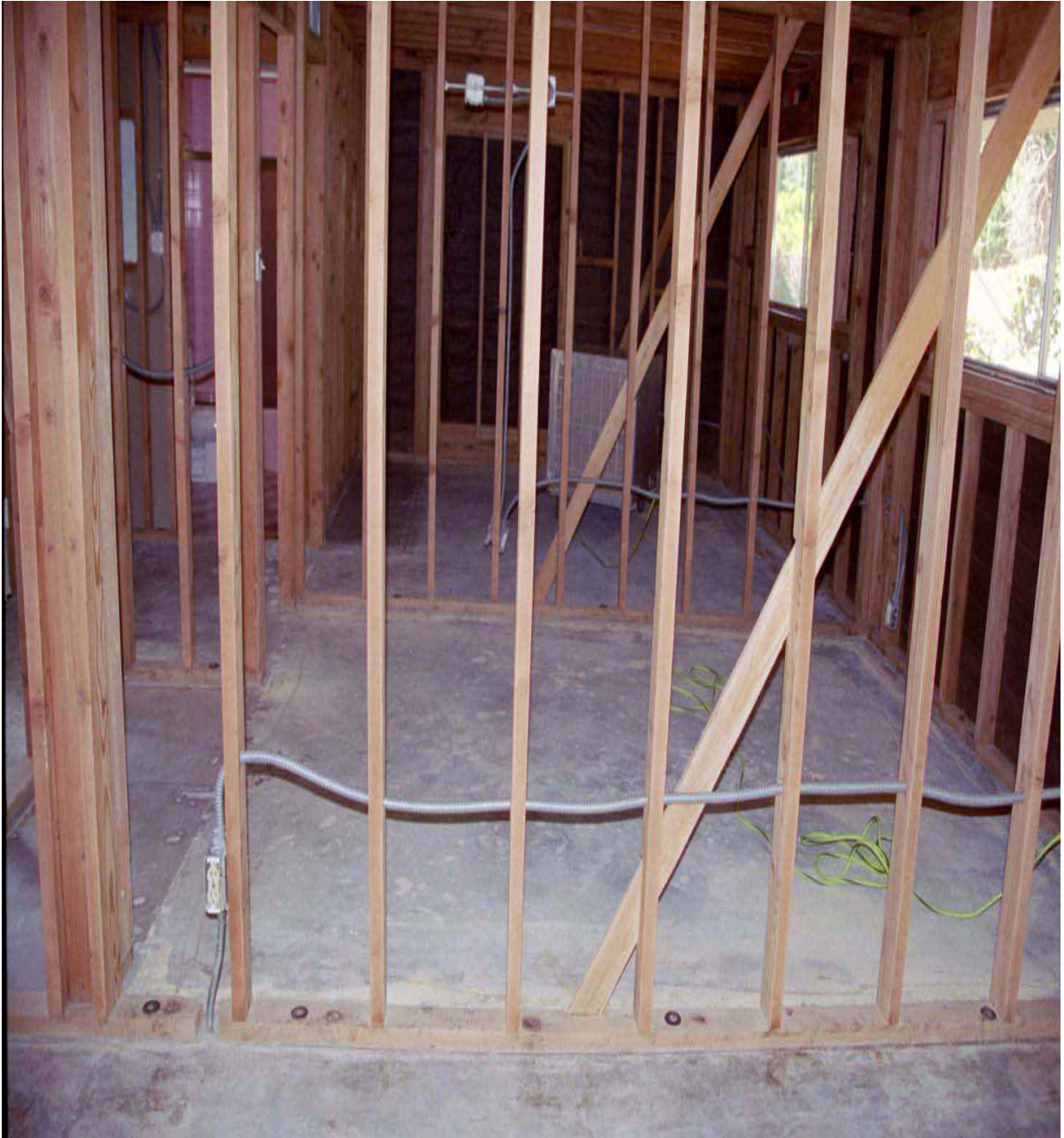
Building framing after mold remediation.
